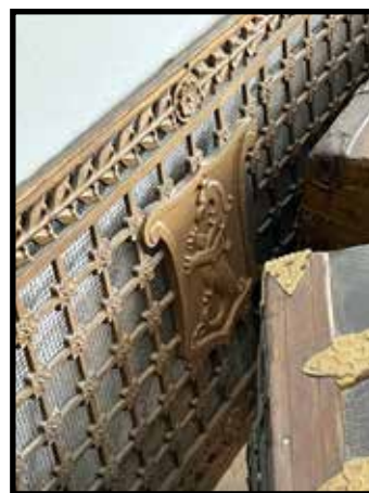
Approx. 11' ornate cast iron air grate St. Louis Fox
