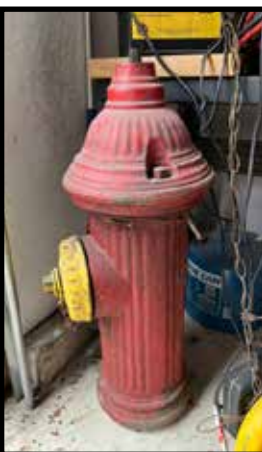
Cast iron fire hydrant
