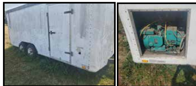
Cargo trailer, tandem wheels with Onan generator, gas motor
